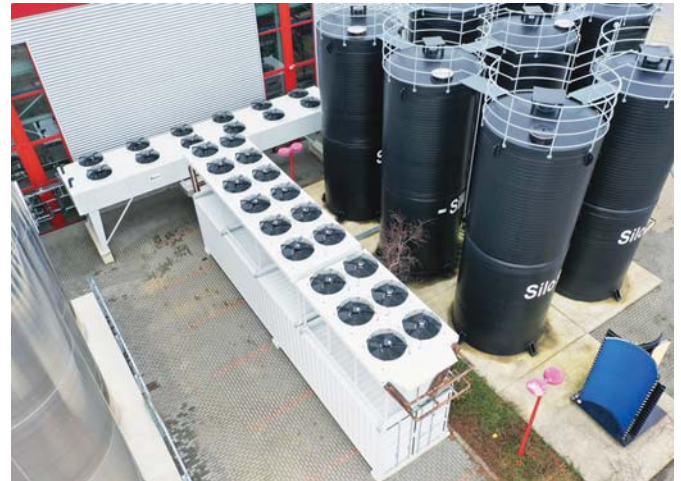
Cooling system container and dry coolers are placed between the new silos on the DRS outdoor area, where they are well protected
