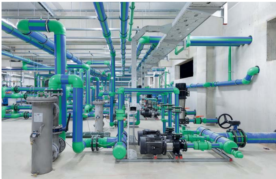
Picture 1: Pipelines from a cooling water treatment system in an industrial plant (Picture: aquatherm)
