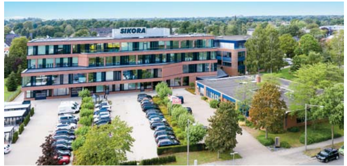
The SIKORA headquarters in Bremen/Germany
