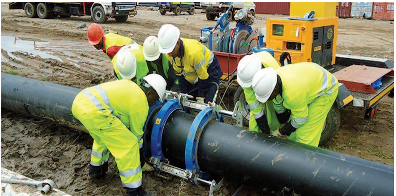
Water pipe installation and welding
