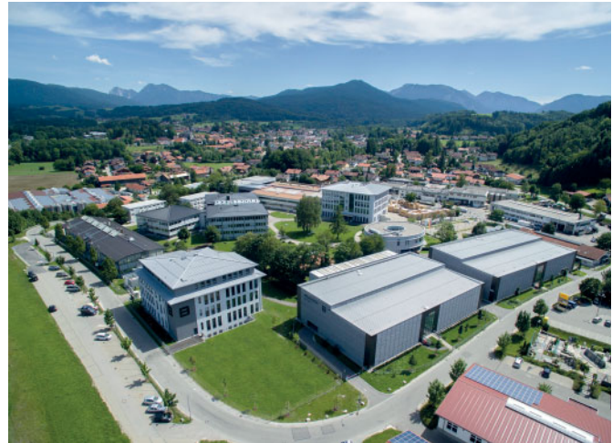
Brückner company premises in Siegsdorf
