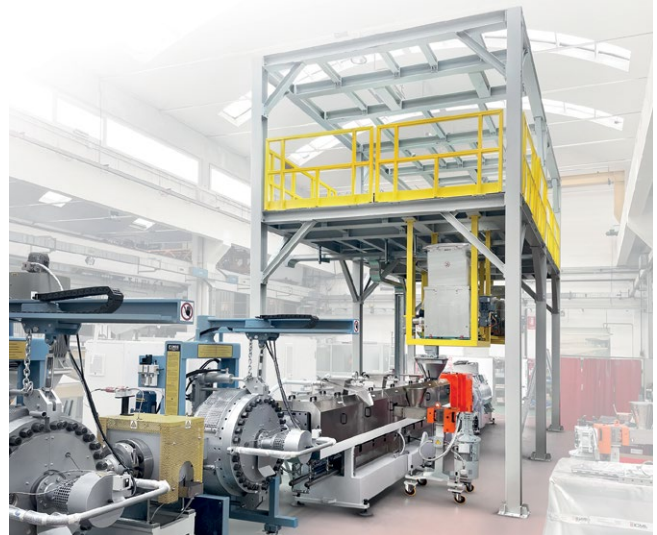
ICMA's line with MCM 110 extruder during installation
