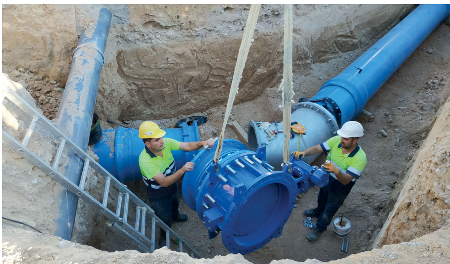
Installation of PVC-O pipes and special pieces in the modernization project of the irrigation area of the irrigation community of the Tajo-Segura transfer of Librilla
