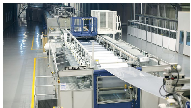
Line Transformation Packages
