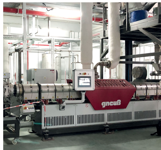
Shot taken during the installation of an MRS extrusion line at Suzhou Shenghong Fiber Co. Ltd, Jiangsu province, P.R.China
