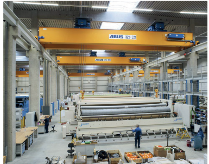
Installation at the Wiehler site
