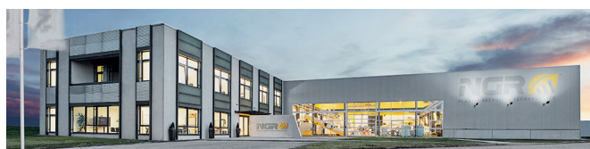
Headquarter Next Generation Recyclingmaschinen GmbH in Feldkirchen a.d. Donau, Austria (Image: NGR)
