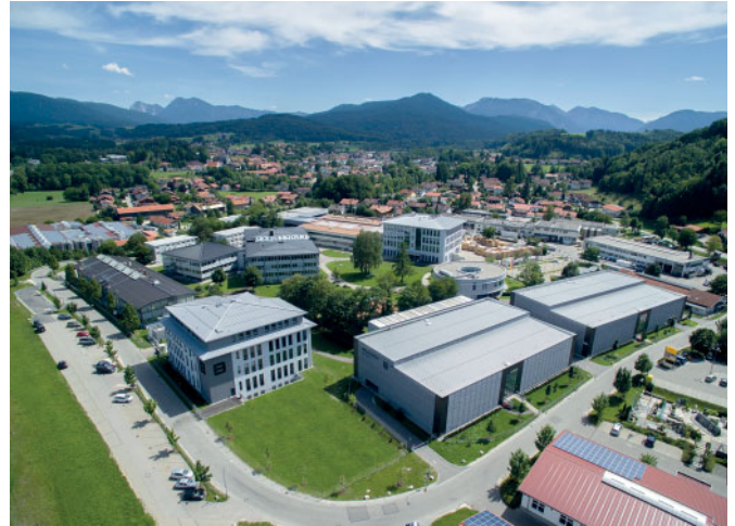
Brückner company premises in Siegsdorf
